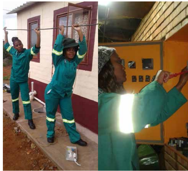
YES learners installing electricity for a household in Warrenton, Northern Cape
