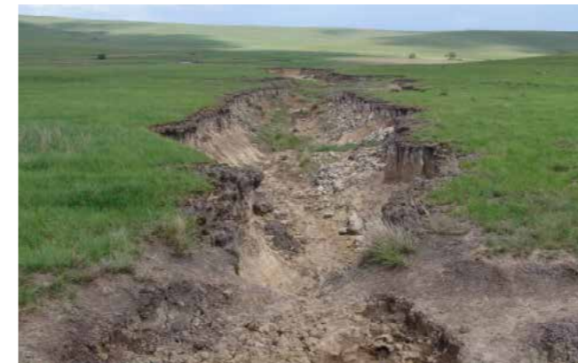
Photo 2: Concentrated runoff discharge from a road, even a path, into a wetland can create a knick, which develops into a gully that grows deeper, wider, longer, and erodes headward. Wetlands incised like this lose their functions of attenuating floods, storing and purifying water, sequestering carbon and supporting biodiversity
