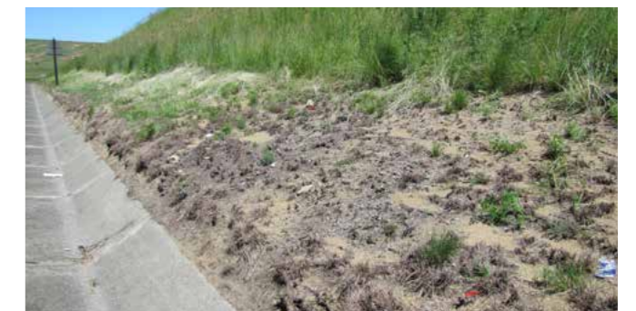
Photo 5: Sometimes they establish grass on the steep cut embankments, then they spray it with herbicide and kill it.
