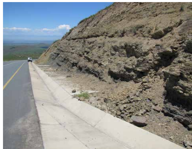
Photo 7b: De Beers Pass not shotcreted 10 years ago
