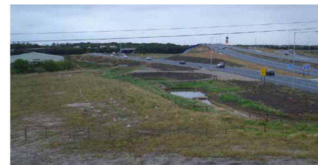
Photo 10: A roadside retention pond receiving dirty road runoff from an interchange in Melbourne, Australia.
