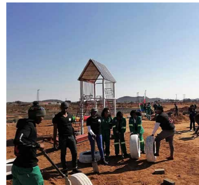
Building a playground in De Aar
