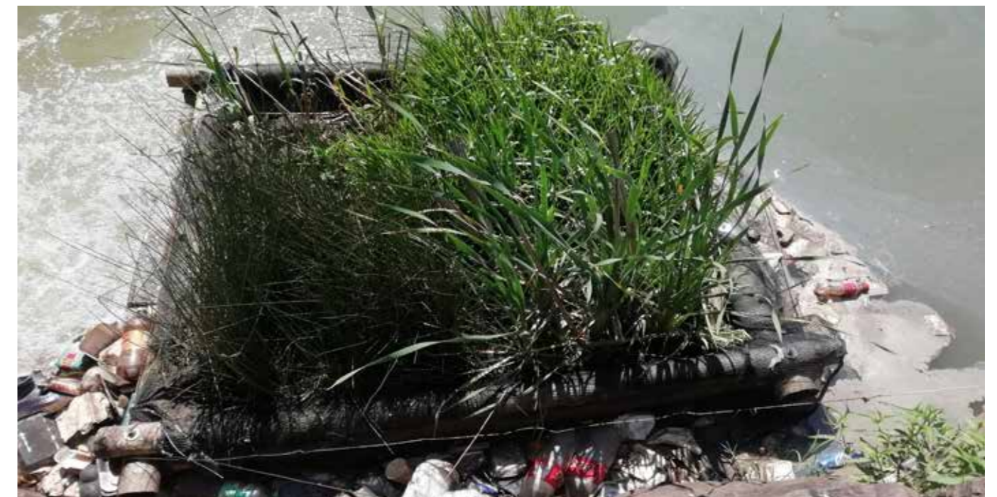
The bamboo floating wetland design installed in the Baynespruit River
