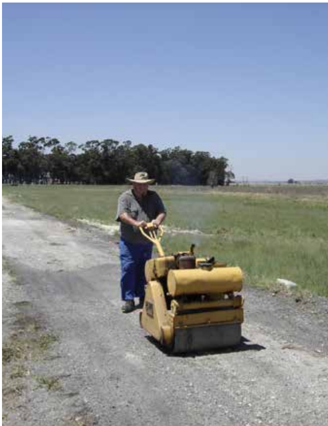
Alan Madden repairing the road at Marievale
